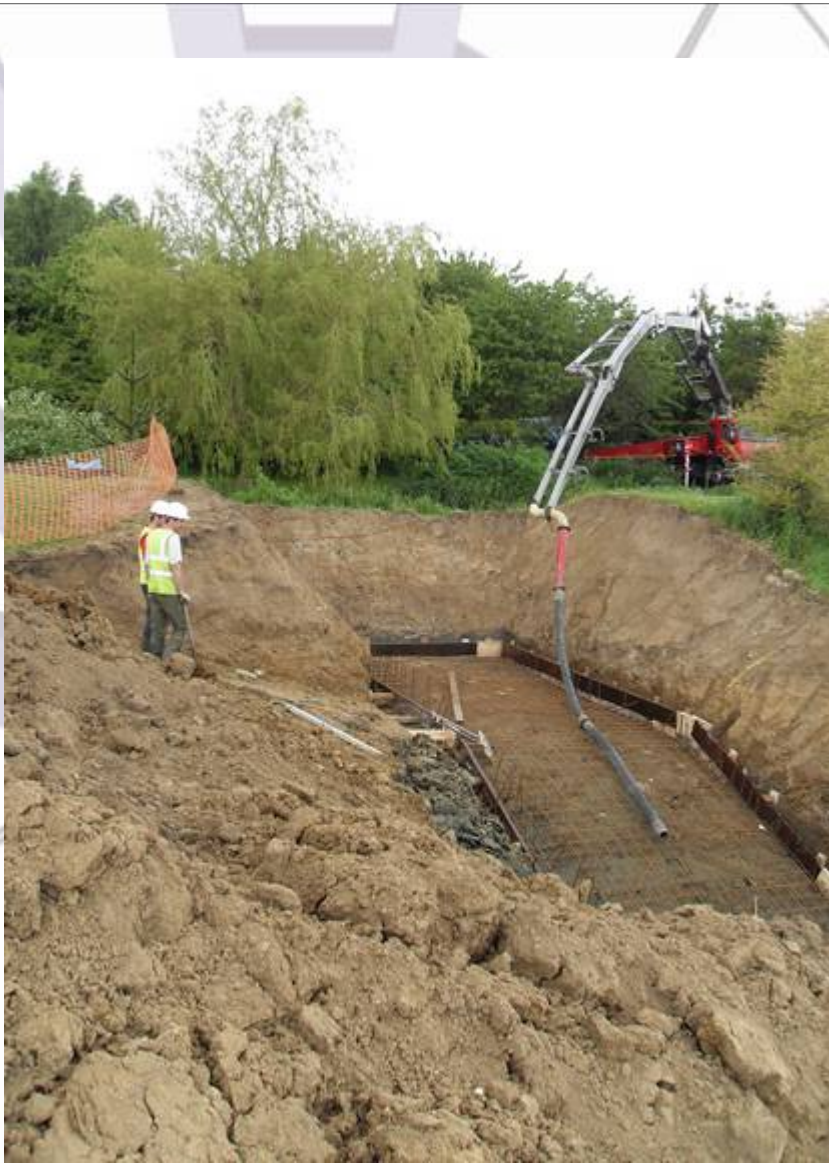
All concrete was pumped to site to overcome access issues
